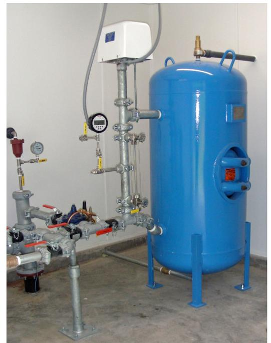
*This pressure tank was installed in a new pressure pump station to maintain good water pressure at a new development at the top of a hill off Elger Bay Road.*
