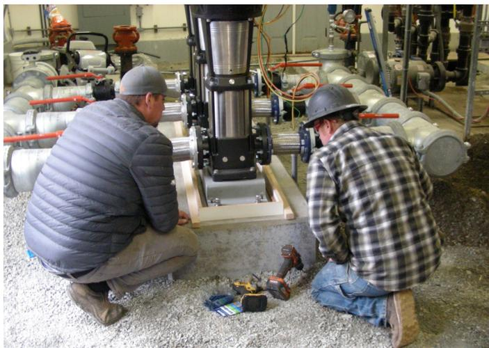
*Workers install new pumps in the expanded treatment plant in early 2020. The CWA treatment plant includes filtration tanks, a chlorine generator, and transfer pumps, all working to remove certain minerals and organic impurities before the water is distributed to your home.*
