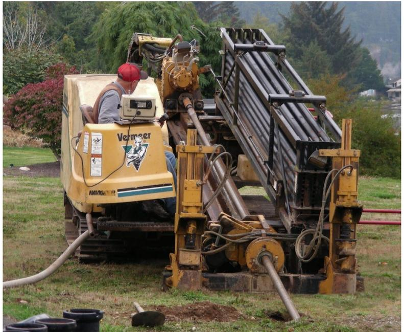
*Willy Bruland of Brulands Drilling and Boring, Inc. is boring a hole under Beach Drive in preparation for the installation of new pipe. The project to replace the corroded 65-year-old pipes in the area started in September and will finish next February.*
