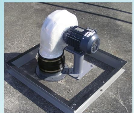
*Forced-air blowers were installed in the three primary water tanks to help resolve the disinfection byproduct (DBP) issue.*
