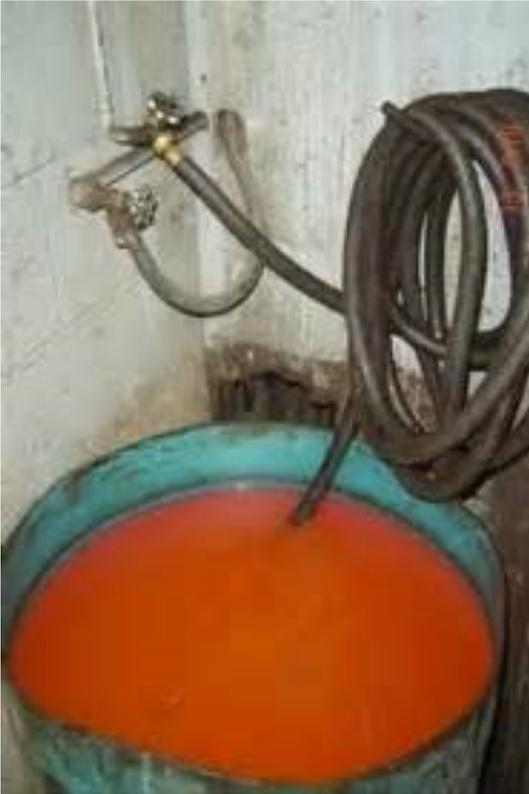
*This hose resting in chemical-laden water could get into a property's drinking supply and then into the CWA public water supply. This will be prevented with the CWA Cross-Connection Control program launching soon.*
